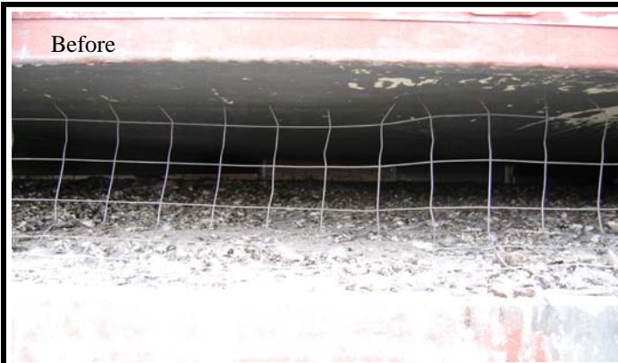
Specialized air systems removes bird droppings from duct work. With the use of air systems (no water), disposal costs are significantly reduced. Once bird wastes are removed; steam is used to sterilize and disinfect work area.
