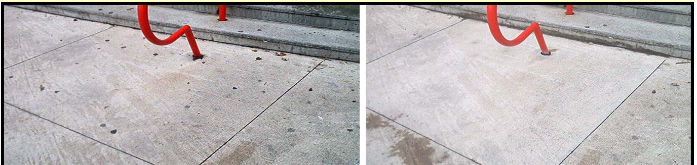
Melts away chewing gum and suctions up the waste leaving concrete free of gum residue and any staining.
